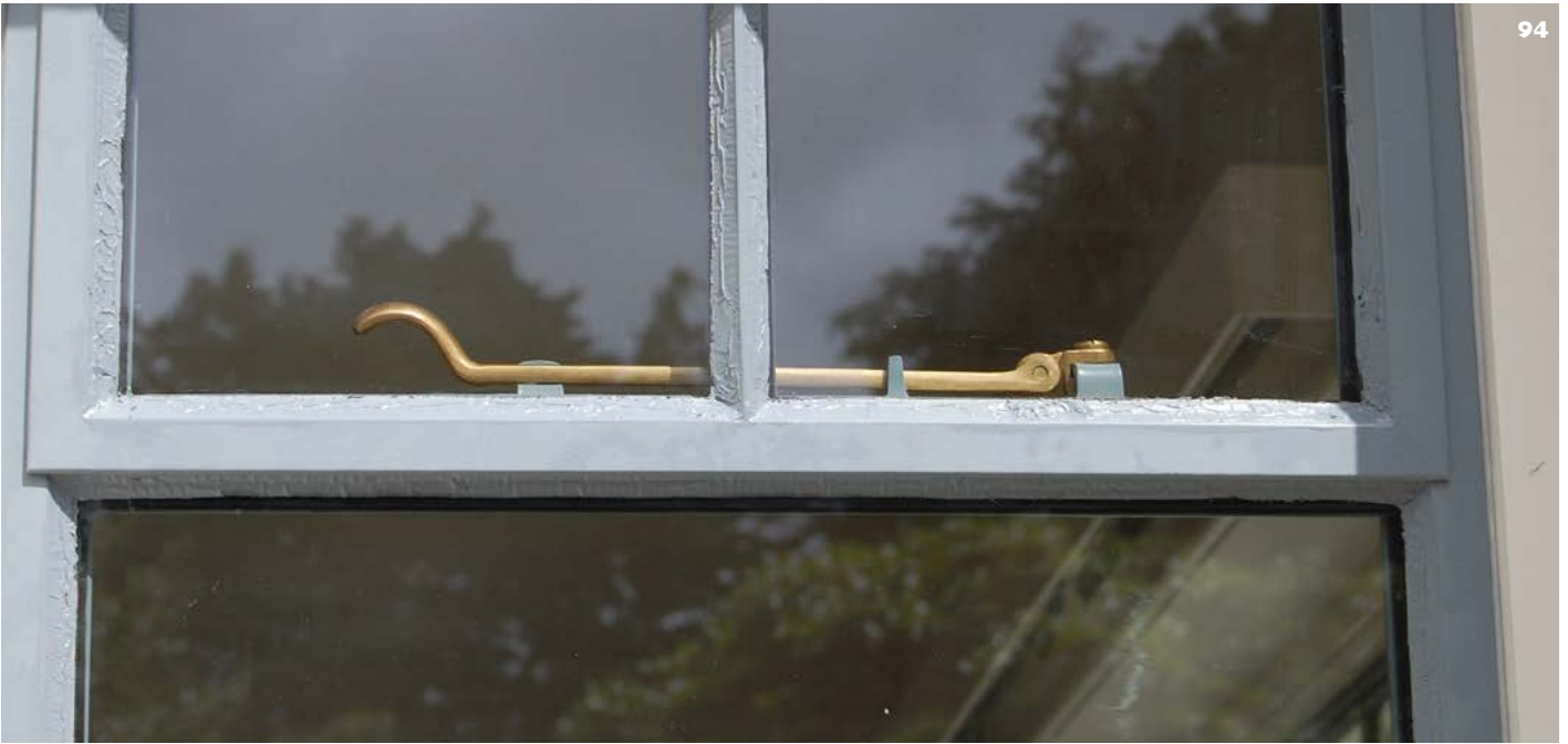
94: The new putty to this steel casement hasn't been allowed sufficient time to cure before being painted. Consequently the paint has blistered.
