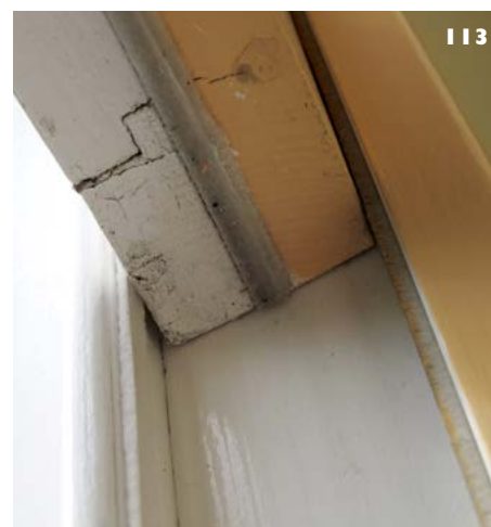
113: A sash window with draught-proofing brushes installed.
