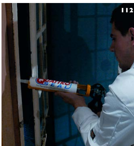
112: Silicone being injected into gaps between the frame and casement to exclude draughts. The casement is first painted with a releasing agent. The silicone is then left to cure with any excess trimmed back.
