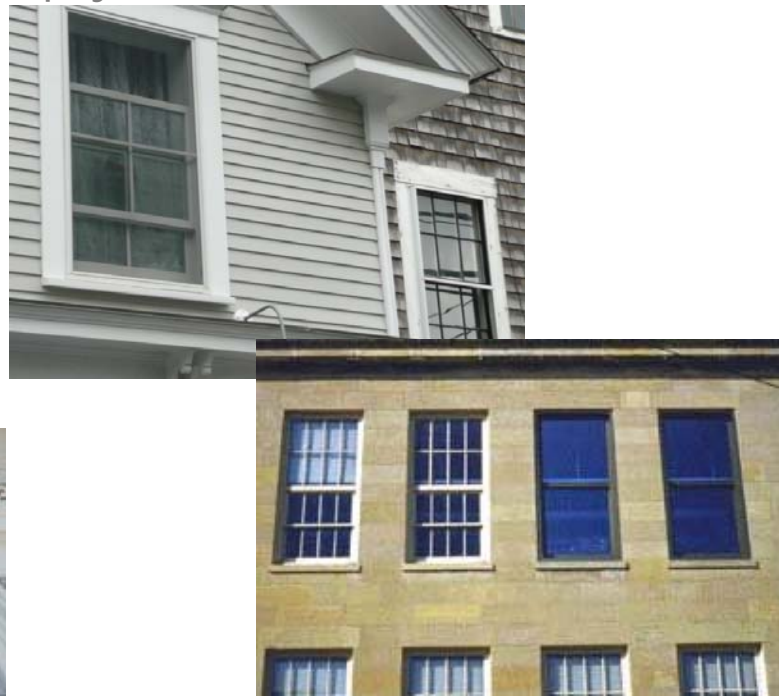
E.g.s where replacement windows do not replicate the original windows in all details.
