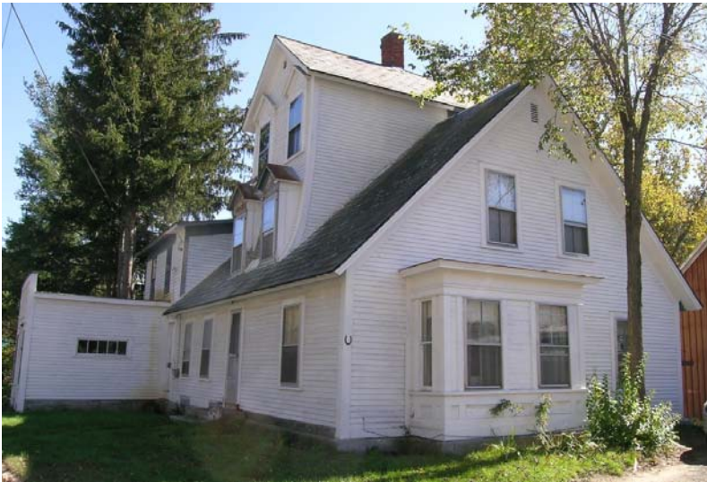
Unusual dormer added to front roof of early Cape.
