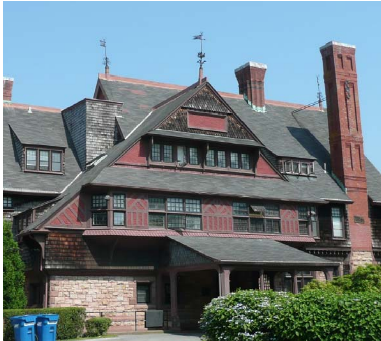
Queen Anne-style house, a style known for use of different surface treatments.
